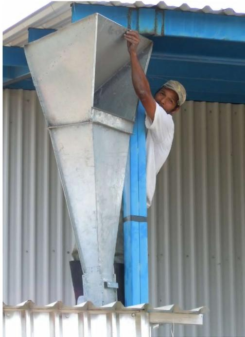
The internet link uses 3G modems provided by local telephone companies used in conjunction with folded horn antennas built by Cafes Sustentables de Mexico. The increased directivity provided by the horn antennas discriminates against multipath interference, reduces fading, and strengthens the signal; thus increasing transferred data rates to usable levels.
